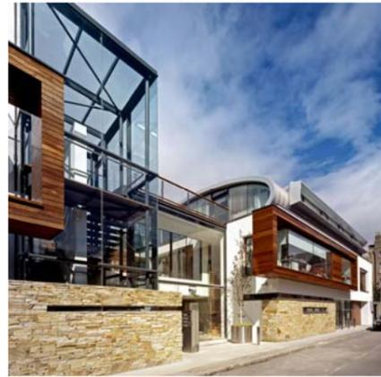
height glazed curtain walling. This steel frame and the landings of the stairs are tied back into the lift shaft walls for stability.
